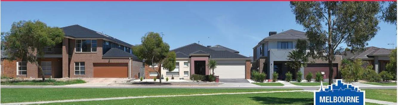
Photo taken at recently Central Equity completed housing estate.
